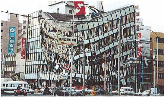
Kobe earthquake, 1995 (Japan)
