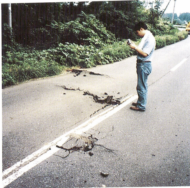
Photo 3 Buckled pavement
