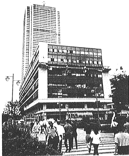
Photo 2 Local collapse at intermediate story of weak-column building
