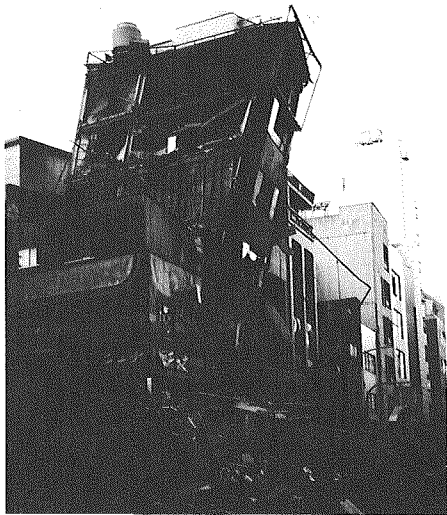
Photo 1 Overall collapse of flexibly jointed steel frame after brace bracing
