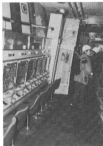
Photo. 6 Interior damage to "Pinball House B".
