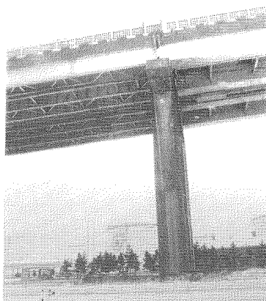
Photo.26 Two different types of girders supported by the pier 12
