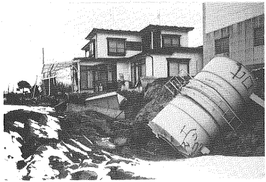
Photo.20 Damage to the reclaimed fill
