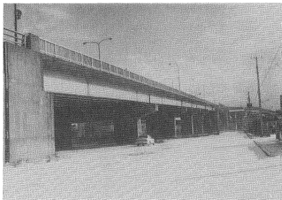
Photo.24 A view of the Hachinohe-Ohashi bridge
