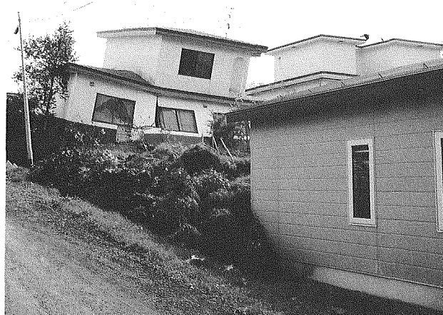
Photo 13 Wooden houses collapsed due to land failure
