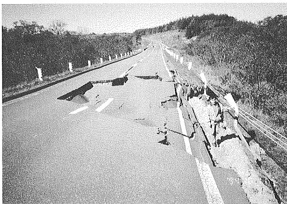
Photo 26 Damage to road diagonally above a corrugated culvert
