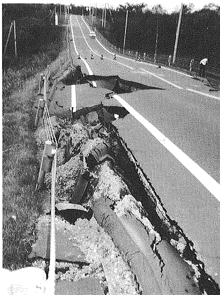
Photo 22 Damage to road at the section between hills
