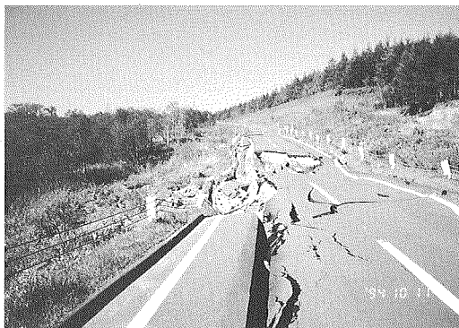
Photo 24 Failure of approach pavement of Shinsei bridge
