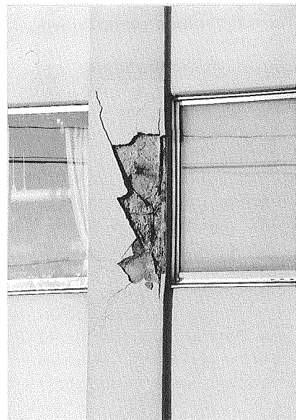
Photo 10 Shear failure of column (Nemuro Hospital)
