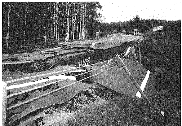
Photo 22 Damage to road at the section between hills
