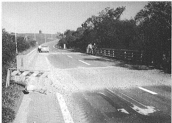
Photo 21 Vertical separation between deck and approach pavement
