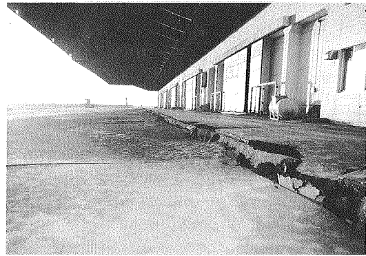
Photo 4 Liquefaction caused similar damage at Kushiro Port (Left: 1993 Kushiro-Oki earthquake, Right: 1994 Hokkaido-Toho-Oki earthquake)
