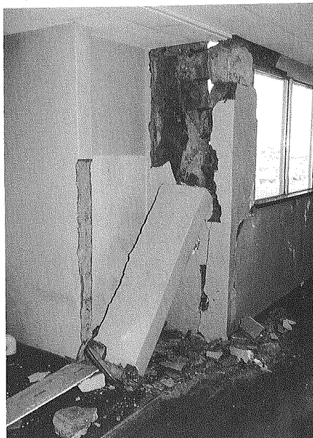
Photo 16 Collapsed nonstructural wall (Koyo Junior High School in Nemuro City)
