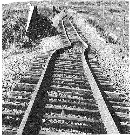
Photo 31 Rails buckled due to subsidence of the embankment at Nemuro Honsen Line
