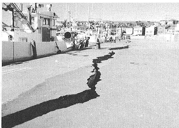
Photo 28 Cracks on quay surface at Hanasaki Port
