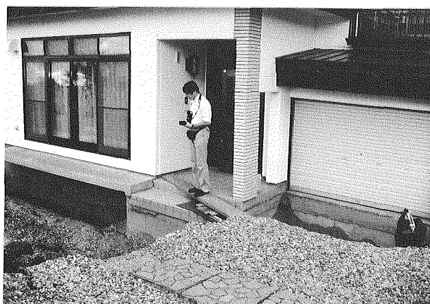
Photo 14 A wooden house with its foundation displaced horizontally by 3.5 m and vertically by 1 m
