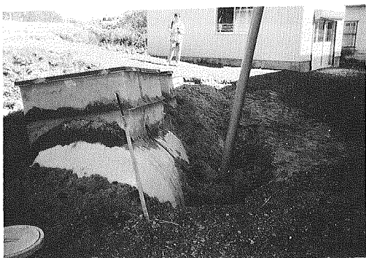
Photo 3 Tank floated up to the surface due to soil liquefaction (Hanasaki)
