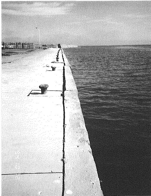
Photo 30 Movement of sheet pile-type quay wall at Bekkai fishery harbor
