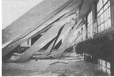
Photo 2: Interior view of the school gym.
