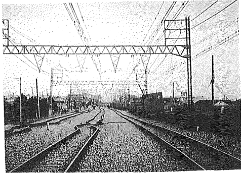
Plate 3 Scene of the crest of the embankment at Tanata site
