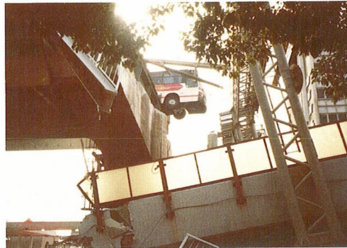
Photo 14 A collapsed section of the Hanshin Expressway in the Great Hanshin EQ. A bus could escape from falling down.
