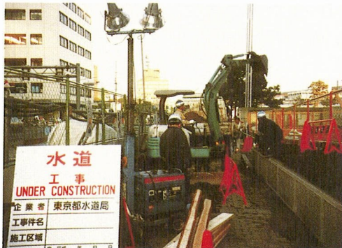
Photo 21 Construction work of water lines in Kobe after the Great Hanshin EQ.
