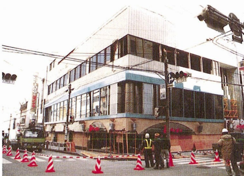
Photo 11 The first story of a pachinco parlor in Hachinohe collapsed in the Sanriku-Haruka-Oki EQ.
