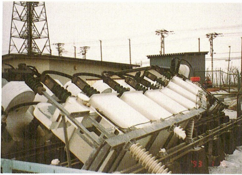
Photo 19 Batteries torn down from the supporting ceramic columns in Kushiyo Substation in the Kushiro-Oki EQ.
