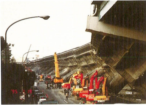
Photo 13 A 500 meter section of the Hanshin Expressway rolled over completely in the Great Hanshin EQ.
