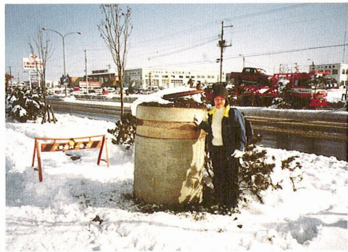
Photo 4 Manholes of a sewage line floated out of the ground due to liquefaction in the Kushiro-Oki EQ.
