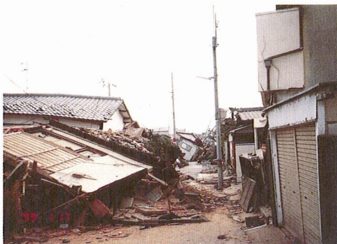
Photo 7 Many wood-frame houses with heavy roof totally collapsed in the Great Hanshin EQ.
