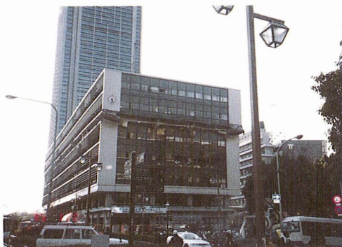
Photo 9 The old building of Kobe City Hall collapsed at a mid-story in the Great Hanshin EQ.
