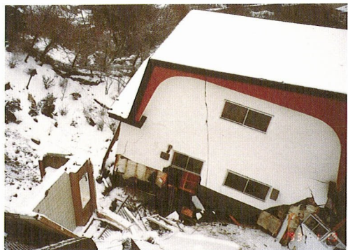
Photo 3 A house slid down a slope in the Kushiro-Oki EQ.
