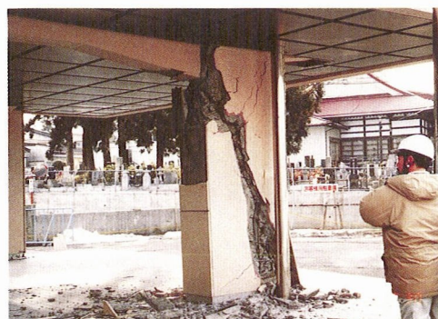
Photo 12 A shear crack developed in a reinforced concrete column of a high school building in the Sanriku-Haruka-Oki EQ.
