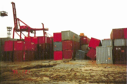
Photo 6 Extensive liquefaction occurred throughout Port Island in the Great Hanshin EQ.
