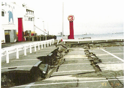
Photo 5 Settlement of pavement with cracks were observed in Hakodate Port in the Hokkaido-Nansei-Oki EQ.
