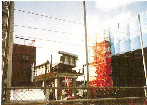
Photo 16 A Sanyo Shinkansen (bullet train) bridge overpassing another railway line collapsed in the Great Hanshin EQ.
