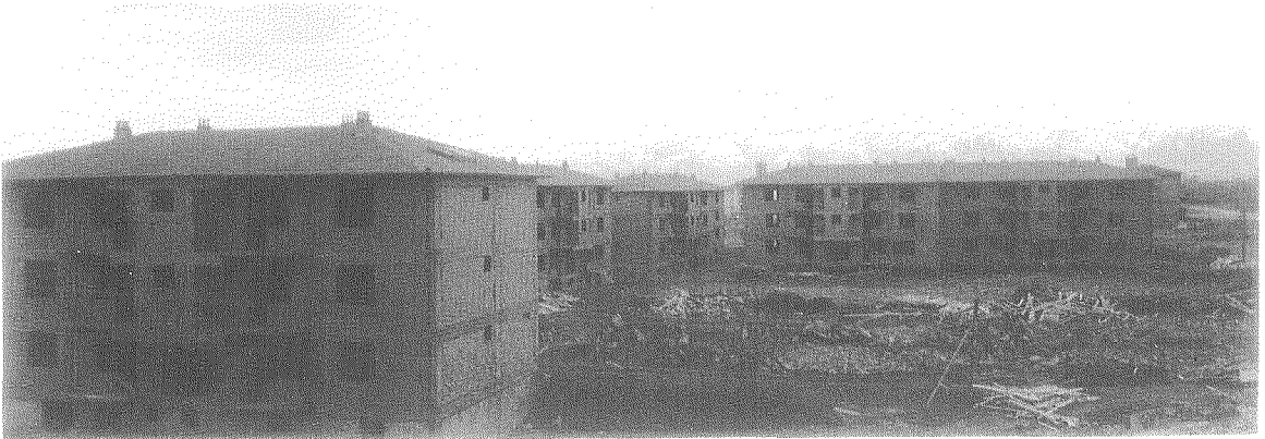
Photo 1: Three-story apartment building under construction in central Yavuz Selim District
