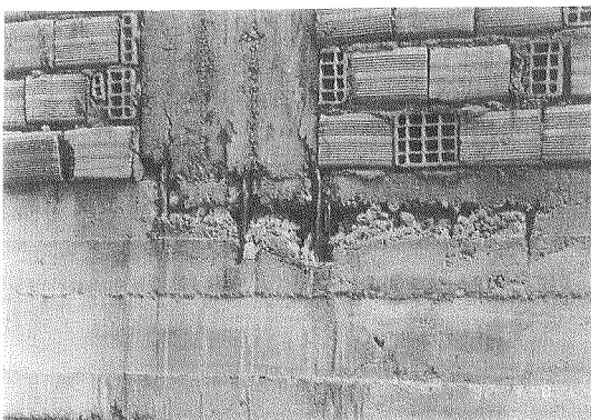
Photo 9: Honeycombs in concrete
