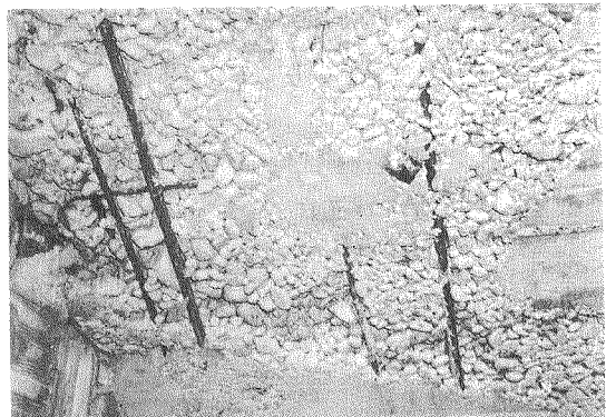
Photo 9: Honeycombs in concrete
