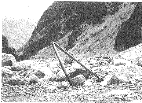
Photo 28 Fallen pole, hit by rolling boulders
