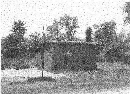
Photo 5 In-place erected clay adobe structure
