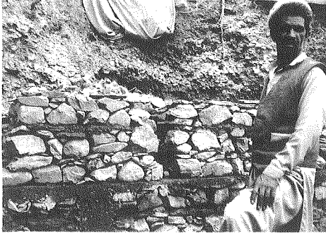
Photo 7 Irregular stones, embedded in mud mortar
