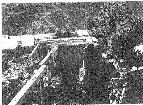
Photo 19 Collapsed houses in Drosh
