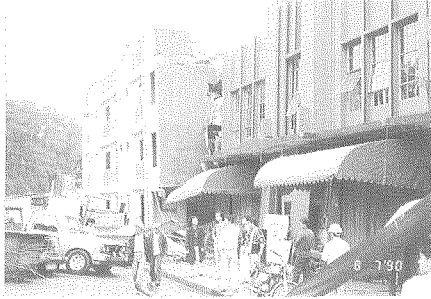
Photo 46 Siesta Inn (left) is leaning forward and is currently being demolished at time this photo was taken (building on the right is Cafe Amapola).
