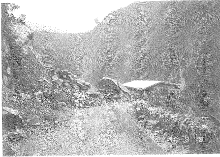
Photo 1 Kennon road blocked by rockslides
