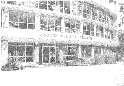
Photo 28 Almost completed repair of Baguio Medical Center
