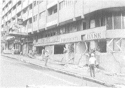
Photo 23 View from Session road of Skyworld building
