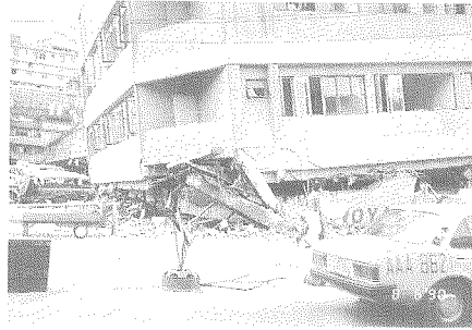
Photo 14 The Royal Inn building moved about 2 meters to the left
