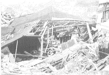
Photo 15 The completely collapsed structure of Aurora Theater
