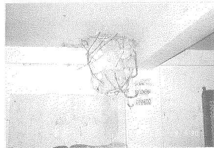
Photo 10 Punching shear failure at the basement of the Commerce building
