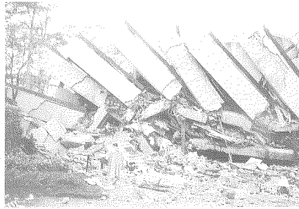
Photo 36 "Pancake" collapse of 11 storey Hyatt Tower building
