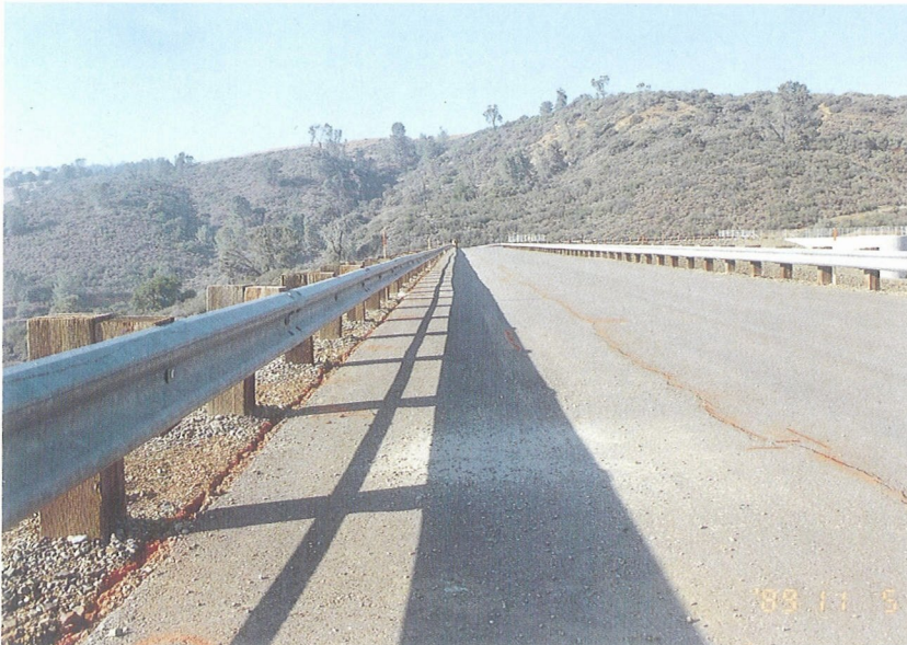
Photo 4. There are about 7 dams in the area within the epicentral distance of 20km. All of them are of fill-type and minor damages on these dams are reported. Longitudinal cracks are running on the Anderson Dam ( \Delta=20\text{km} ) where the maximum horizontal acceleration was 0.43g on the crest and 0.23g at the downstream recorder site.
