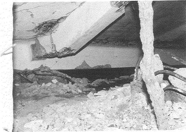
Photo 7. Crushed column of same building
