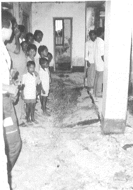
Photo 9. Damaged floor due to soil liquefaction
