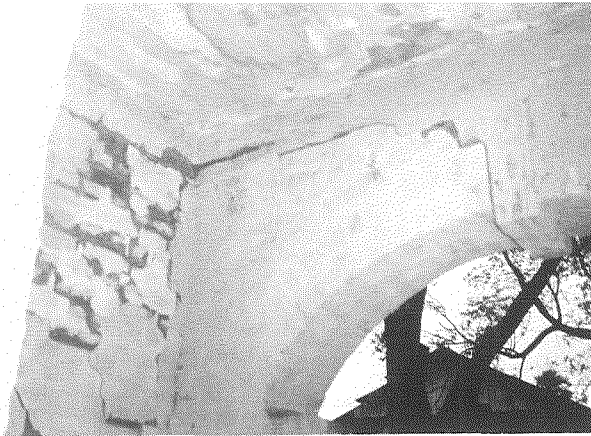
Photo 5. Cracked arch of same building
