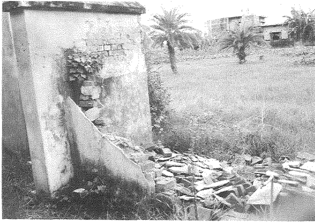
Photo 1. Collapsed boundary wall of Girls School, undamaged RC house in back view (Dharbhanga)
