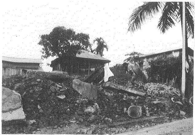
Photo 16. Collapsed masonry dwelling, intact tin roof house in backview (Dharan)
