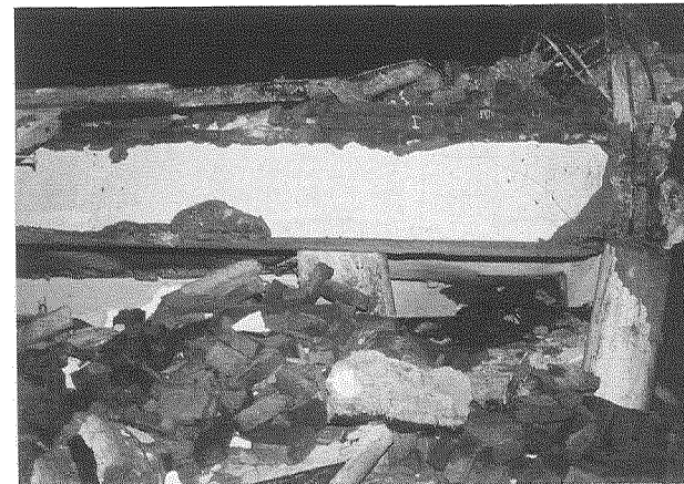
Photo 8. Undamaged beams of the same building
