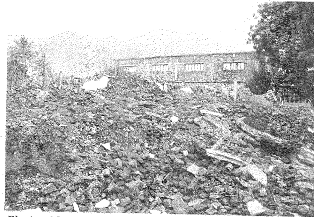
Photo 18. Collapsed masonry of school building, intact RC frame in back view (Dharan)
