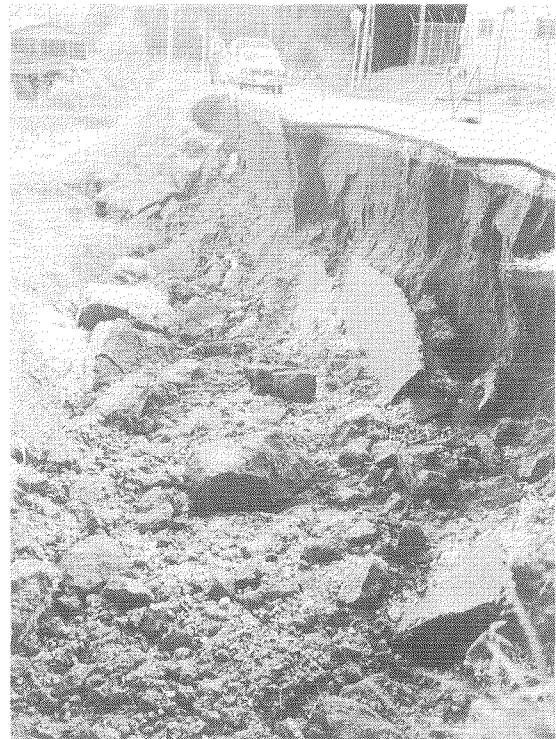
Photo. 13 Collopse of a shoulder of road in Mobarra city
