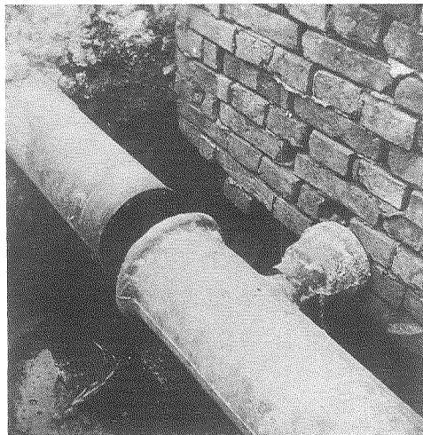
22. Damage of Castiron Pipe at Wall Crossing
