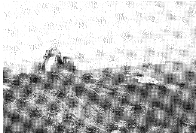
Photo. 7 Damaged Embankments Under Repairing at Yamazaki
