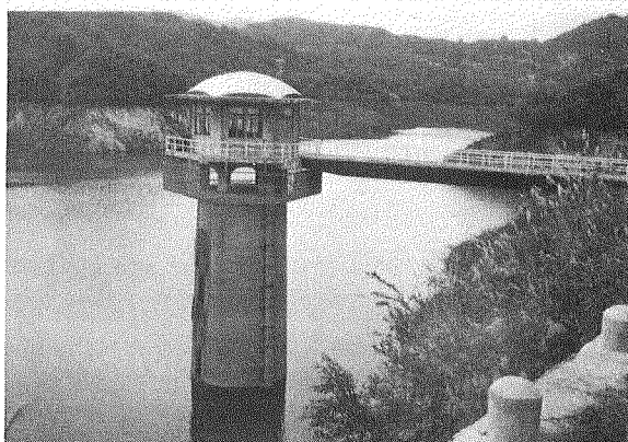
Photo. 3 Intake tower of the Ainono Dam
