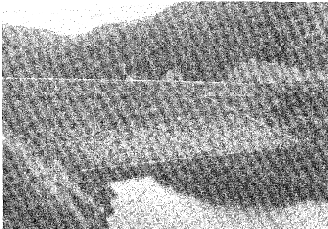
Photo. 1 View of the upstream side of the Ainono Dam
