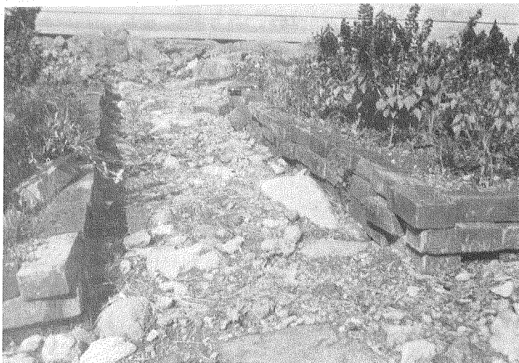
Photo. 4 Slip of the brick laying, the Sanmata village
